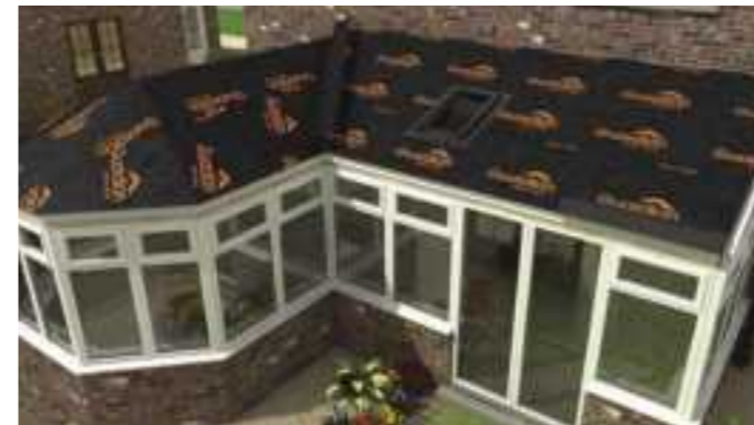
Breathable waterproof membrane is laid over the plywood and secured in place.
