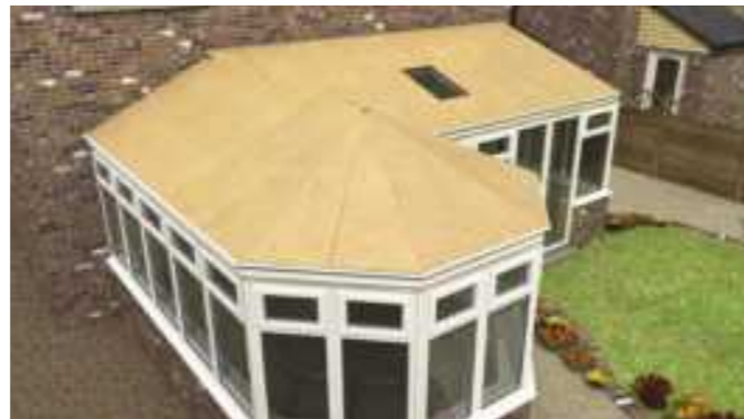
Exterior grade plywood is fixed to the rafters.
